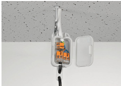
Pendant light connection in a suspended ceiling
